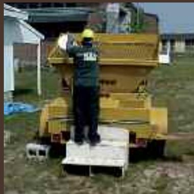
Figure 2: Loading Hopper of the Press with Soil
